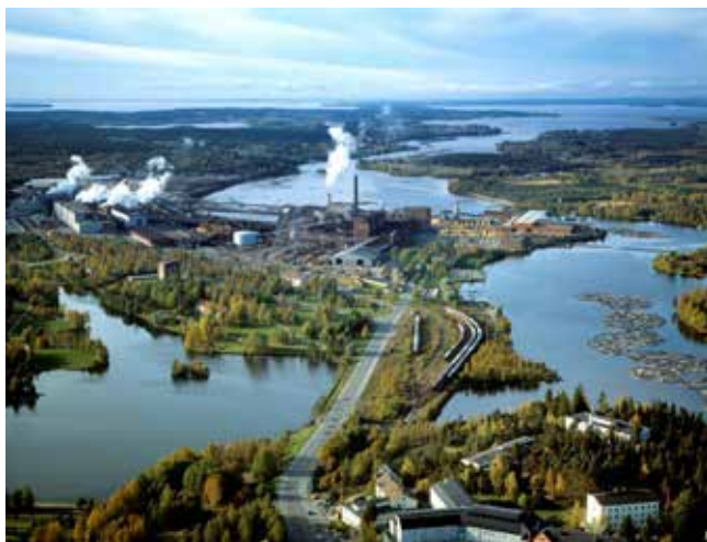
The CSC Kajaani Data Center (site of SDC-FI hardware), on the left, is located in a former paper mill.
